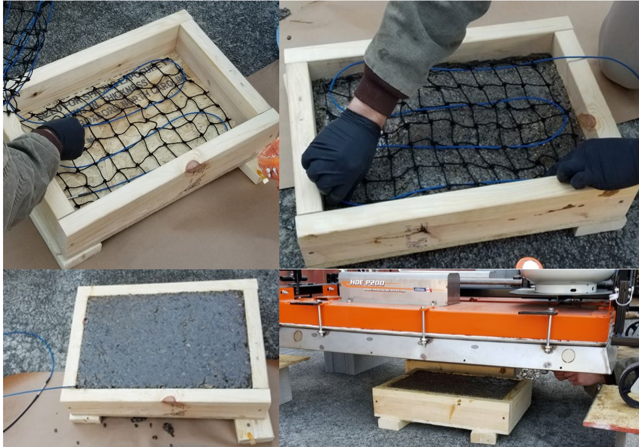
Figure 4. Incorporation of fiber optic within repair patch
